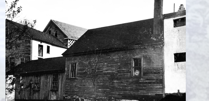
Views of the Faulkner mill buildings in 1969.
